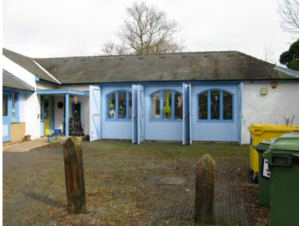
Former stables and laundry to the north of the Hall
