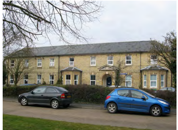
St Peter's House – the second school, on the north side of Church Lane
