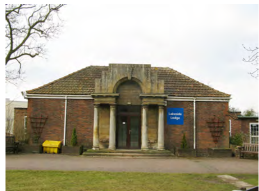
The Simms Woodhead Building (Lakeside Lodge)
