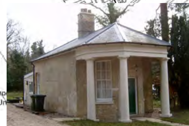
Lodge to Papworth Hall Main Entrance
