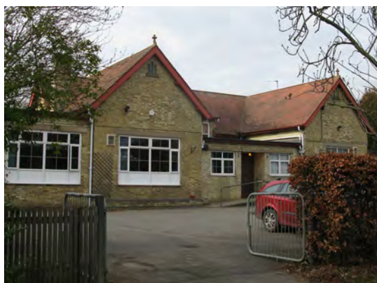
St John's Hostel, the 1901 school, on the west side of Ermine Street south
